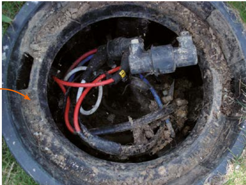
K199 - Installation in a pit
