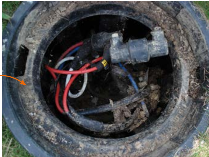
K199 -Installation in a pit
