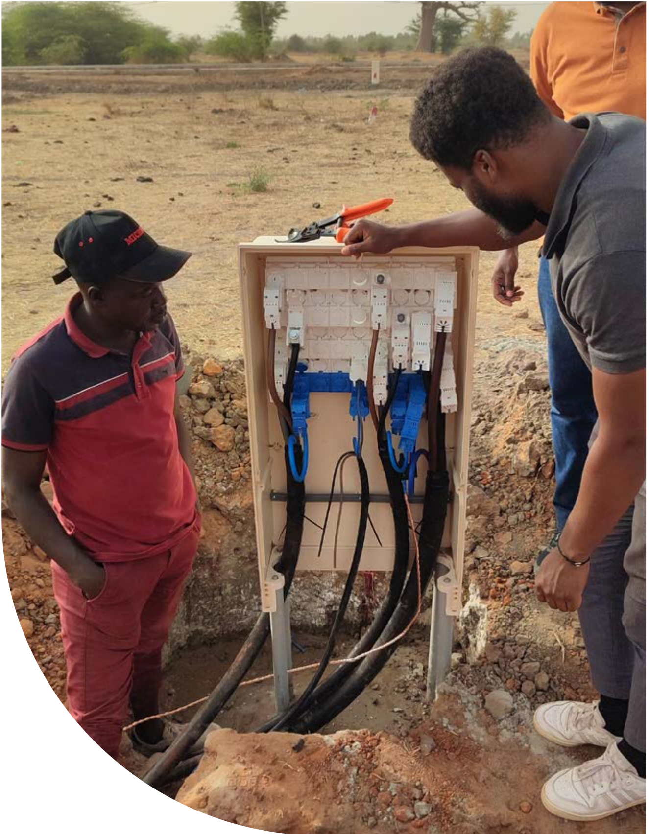
Installation of REMIC cabinet - Senegal
